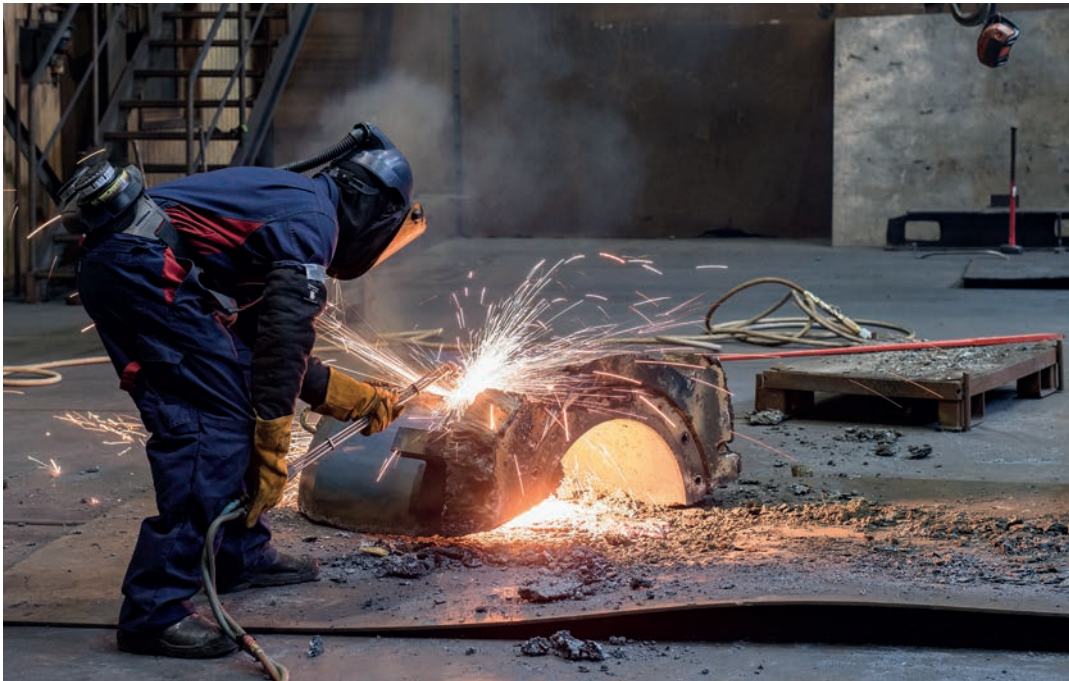
Segmentation of waste local to generation (image courtesy EDF/Cyclife)
