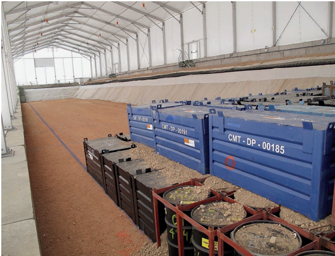
Very low-level waste disposal cell at Enresa's El Cabril facility in Córdoba, Spain (image courtesy Enresa)
