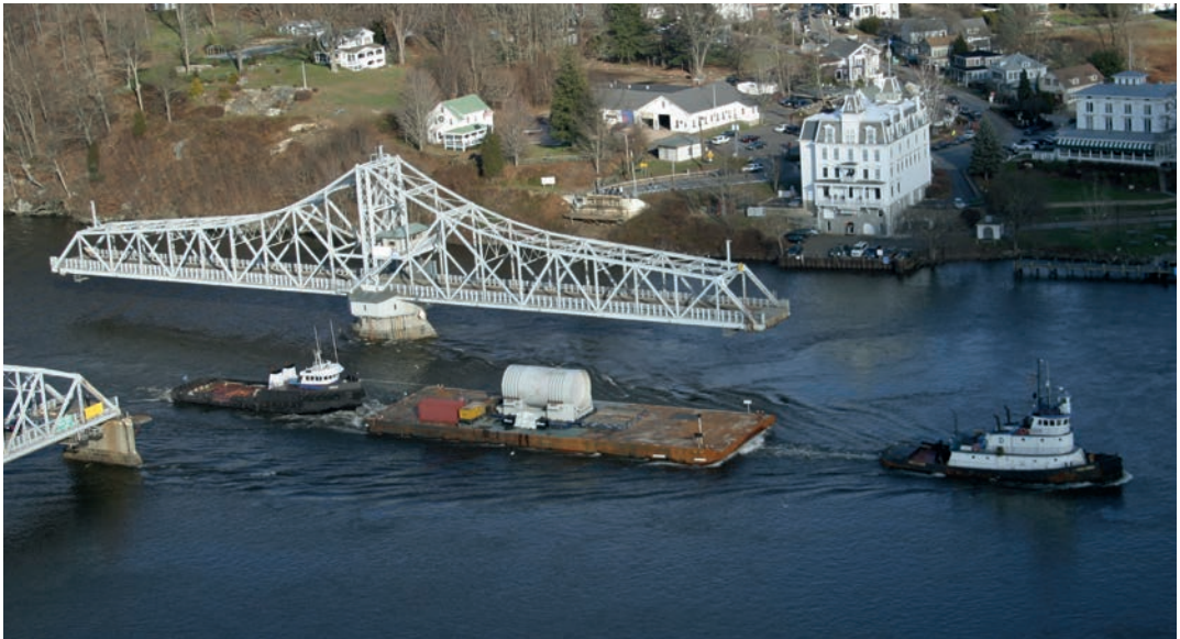
The 619 MWe Connecticut Yankee PWR at Haddam Neck operated from 1968 until 1996, and was decommissioned in 1998-2007. The image shows the Connecticut Yankee reactor pressure vessel shipment by barge during decommissioning (image courtesy Connecticut Yankee)
